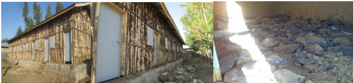
The front and rear view of Teachers Residence and partial view of a room with filled stone
